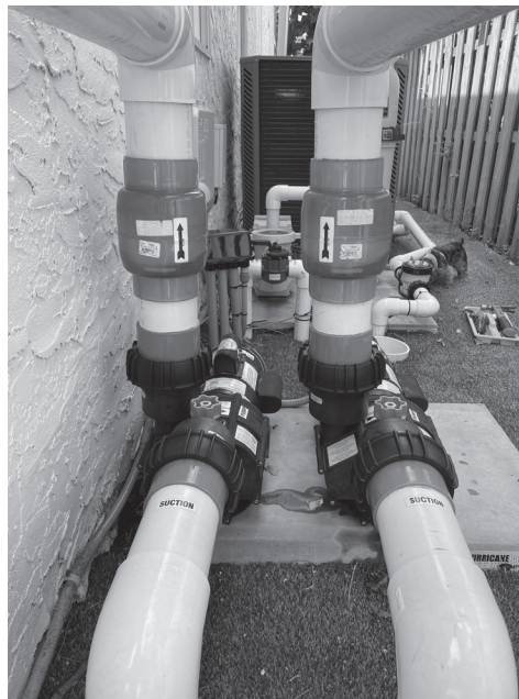
Figure 8 Check Valves Installed for a Package D ( three jet & 2 pump system)
